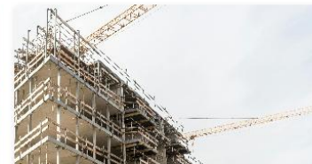
Construction of Buildings
